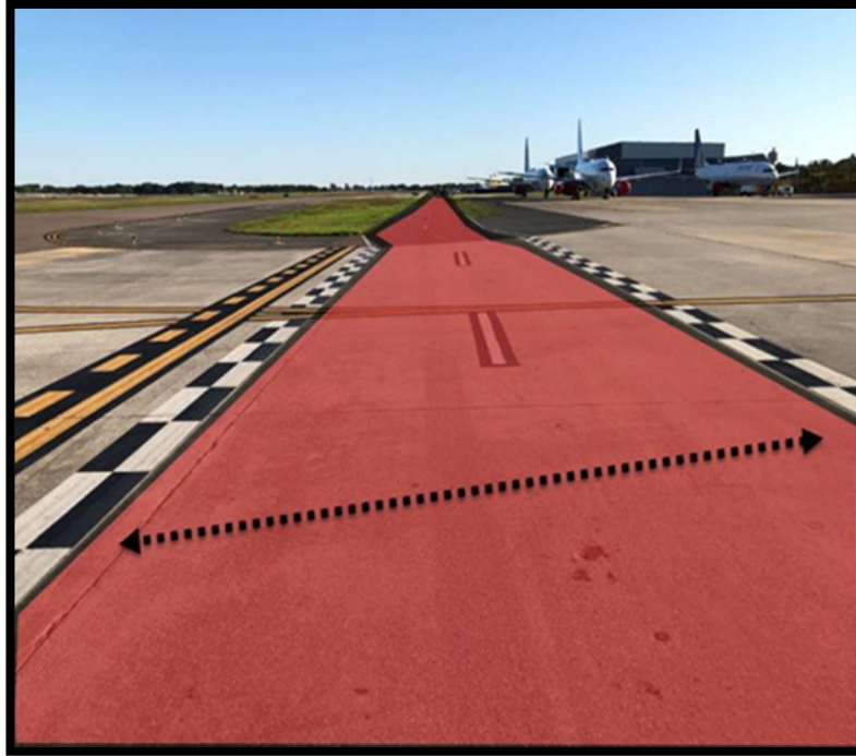
Apron Service Road (Red shading added to delineate)
