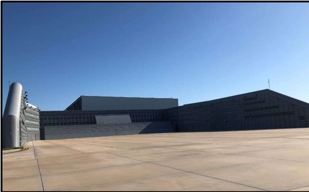
The Maintenance Run-up Enclosure is also commonly referred to as The Hush-House.
