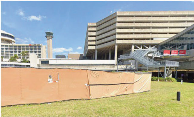
Photo 3: George Bean Parkway, looking east
