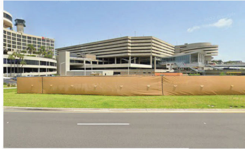
Photo 2: George Bean Parkway, looking south
