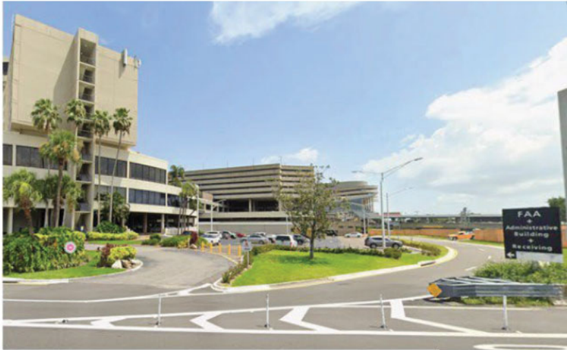
Photo 1: George Bean Parkway, looking south
