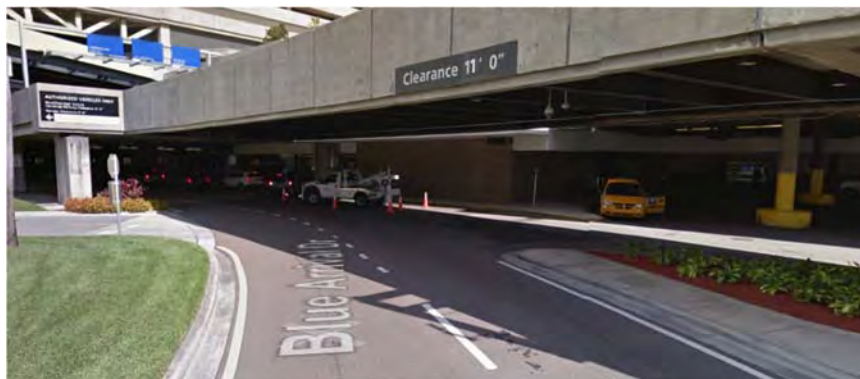
Figure 5.88 Existing Curbside Vertical Clearance
