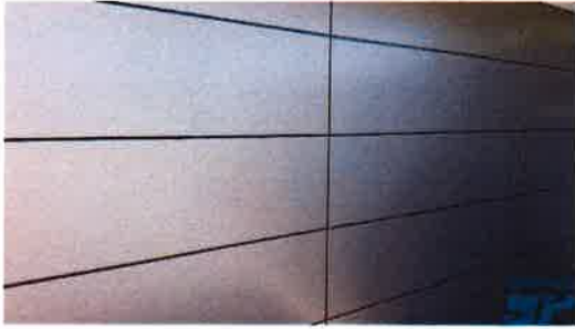
ACM - Aluminum Composite Material: - Soffits - Canopy Trim
