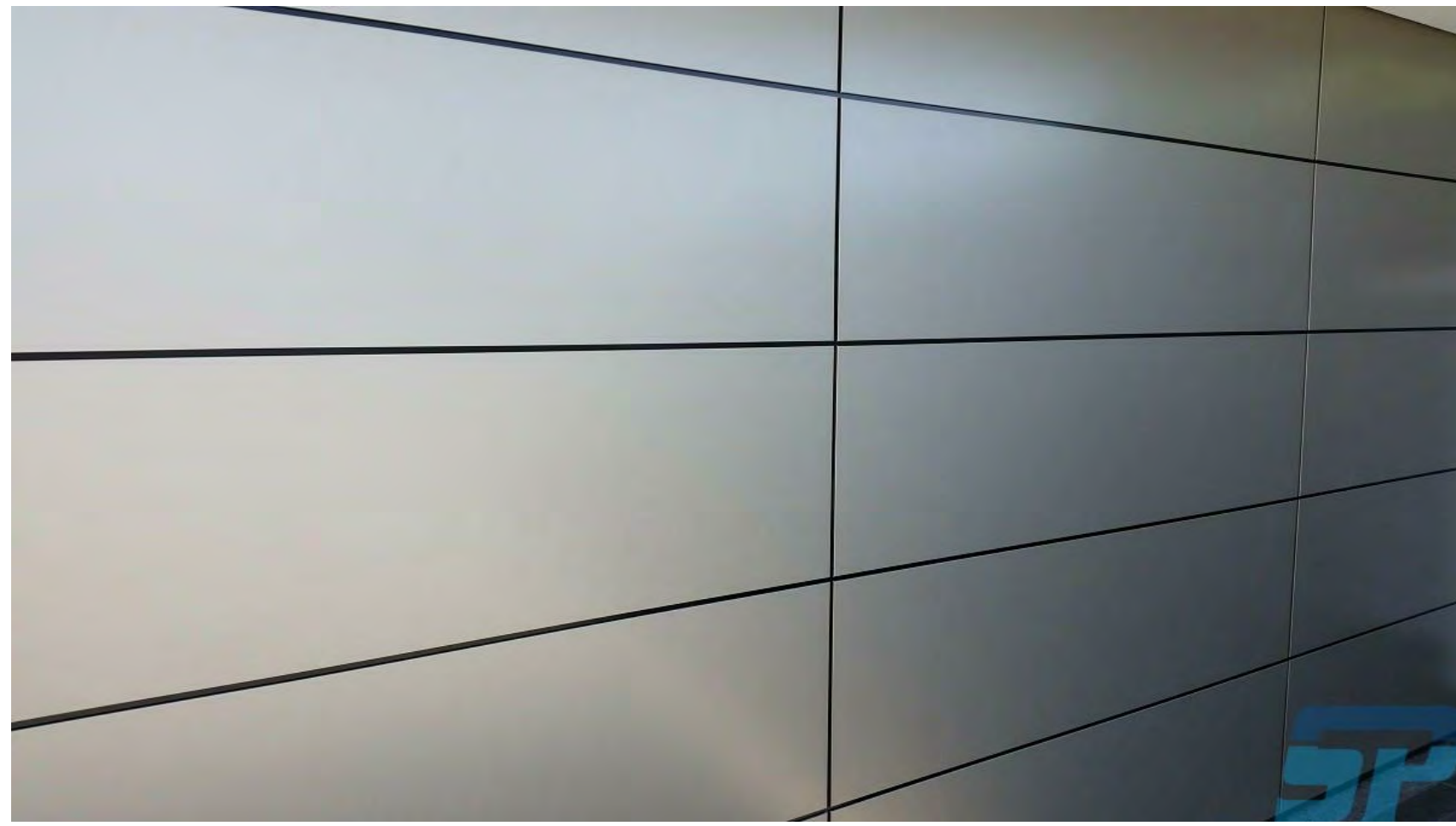
ACM - Aluminum Composite Material: - Soffits - Canopy Trim
