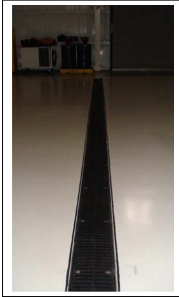
SITE PHOTOGRAPH: INTERIOR FLOOR DRAIN
