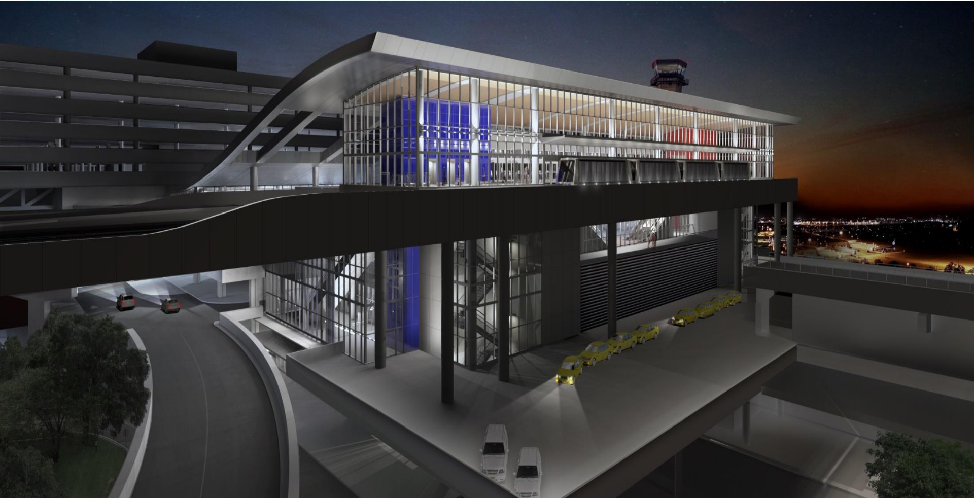
Main Terminal APM Station – Northwest View
