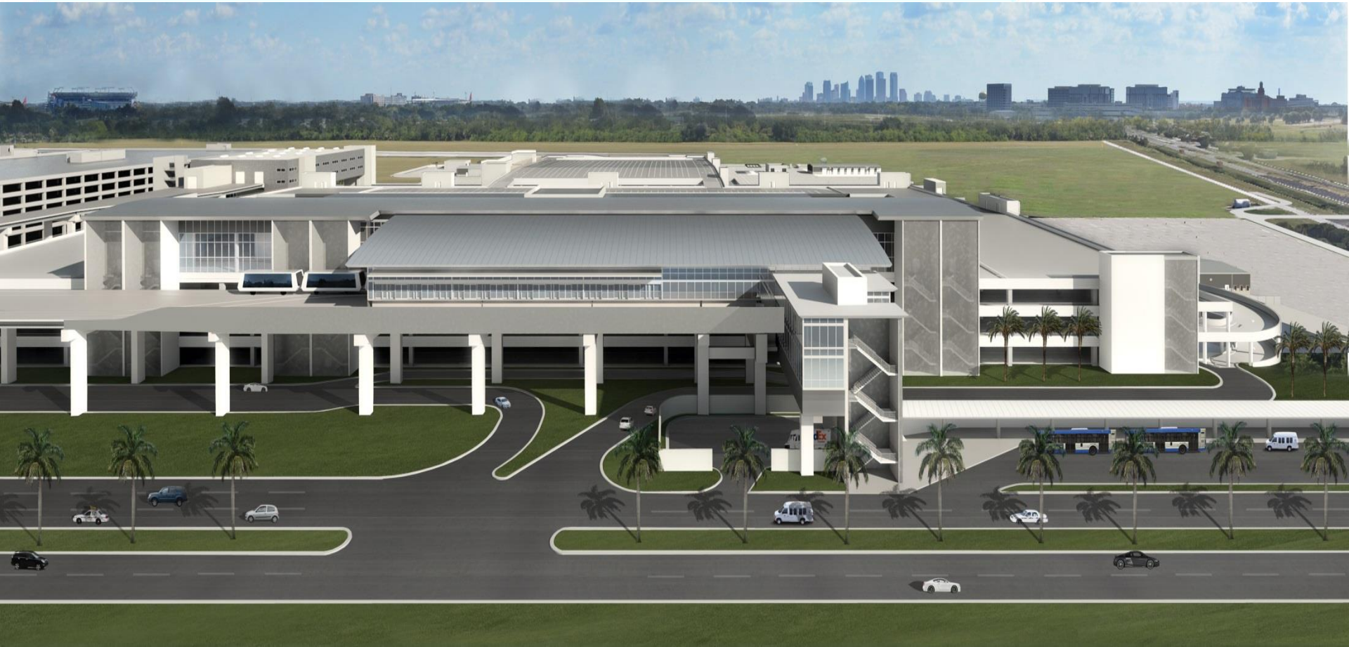
Exterior East View
