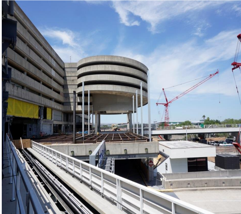
East Transfer Level Expansion
