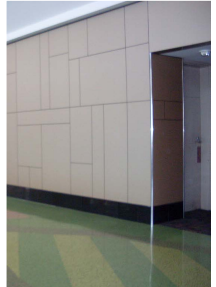
Typical walls and terrazzo floor: Base and floor conditions are to be maintained.
