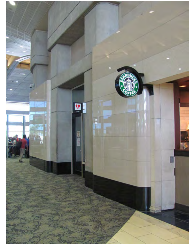
Typical concourse fixed element façade: Polished soft neutral porcelain ceramic panels. These hold the space and yield much freedom for concessionaire insertions to be colorful, textural and saturated.
