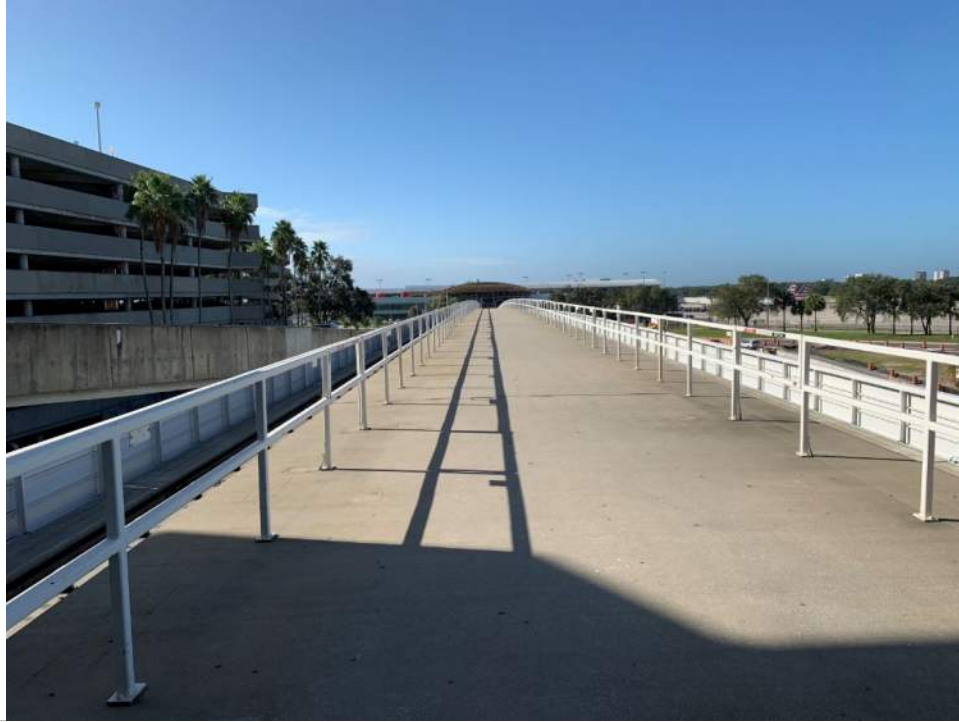
Photo 9 – Overview of Airside F Guideway walkway.
