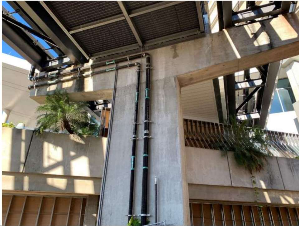
Photo 11 – Overview of Airside F Guideway from below.
