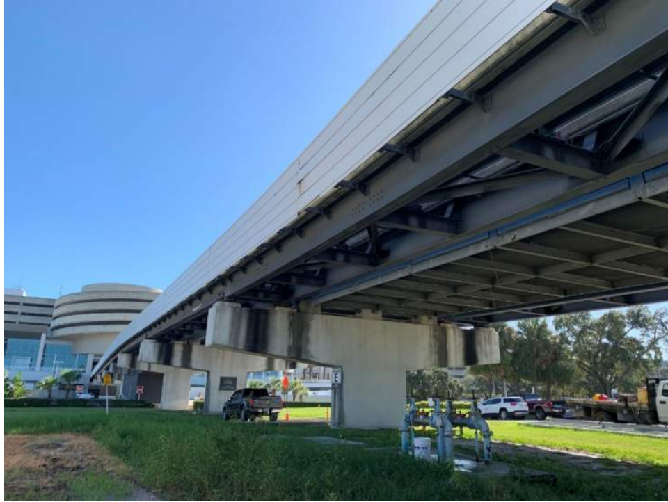
Photo 7 – Overview of Airside E Guideway from below.
