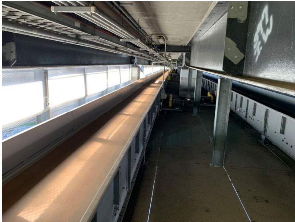
Photo 12 – Overview of Airside F Guideway baggage area below walkway.
