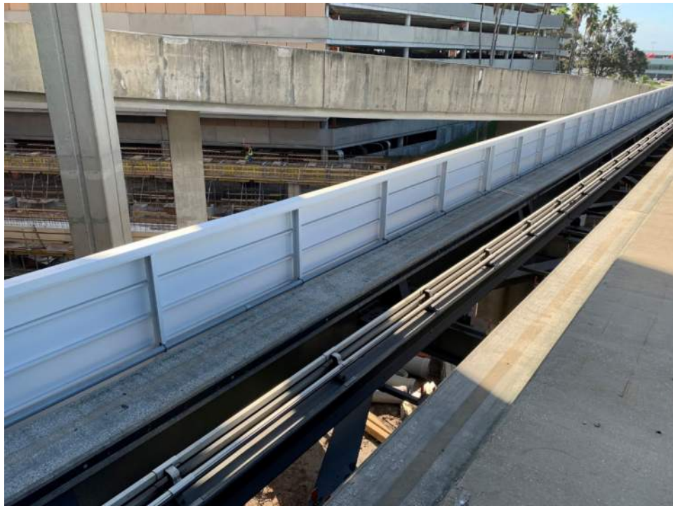
Photo 10 – Overview of Airside F Guideway running surface.
