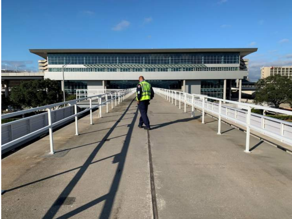
Photo 1 – Overview of Airside A-Sort Guideway walkway.
