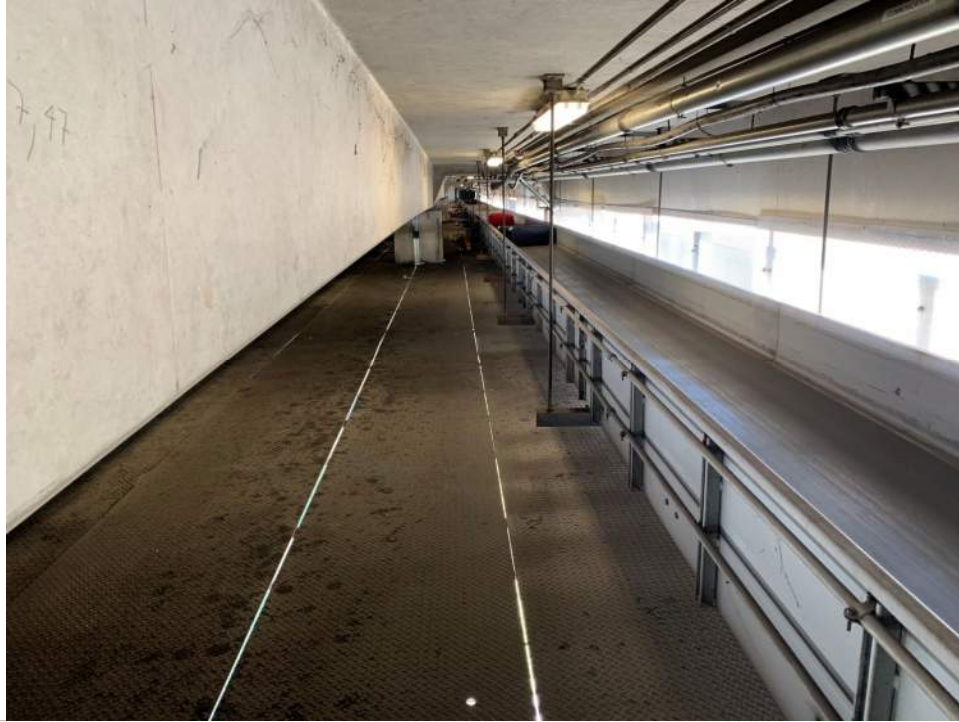
Photo 3 – Overview of Airside A-Sort Guideway baggage area below walkway.
