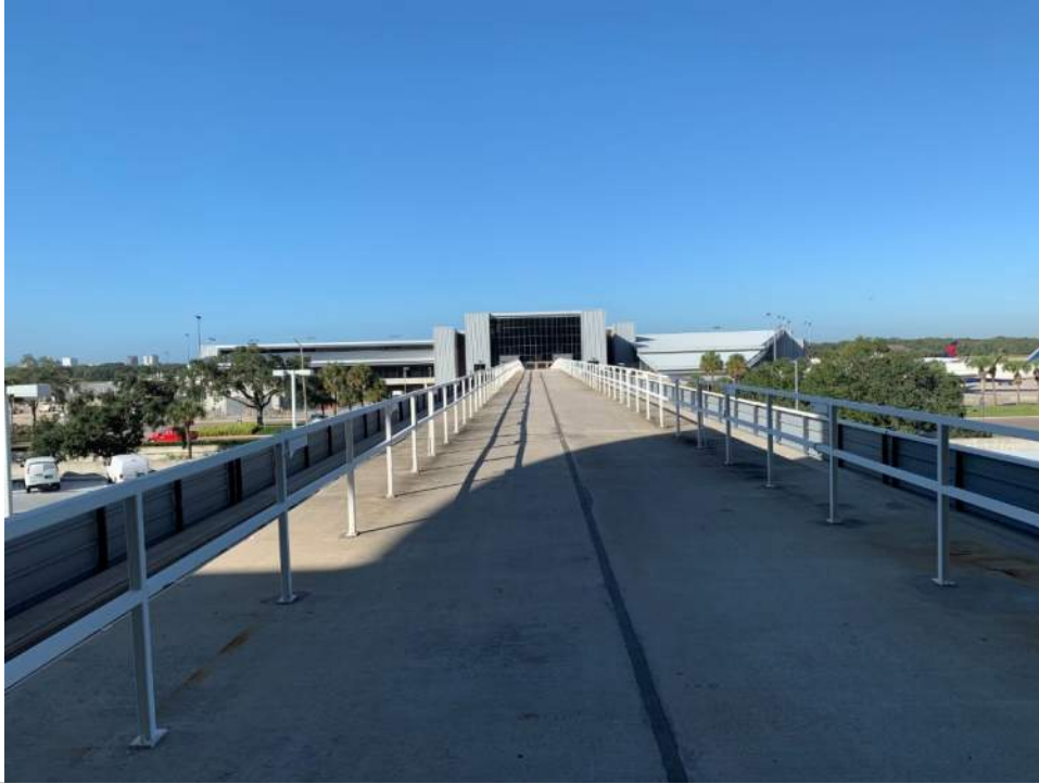
Photo 5 – Overview of Airside E Guideway walkway.
