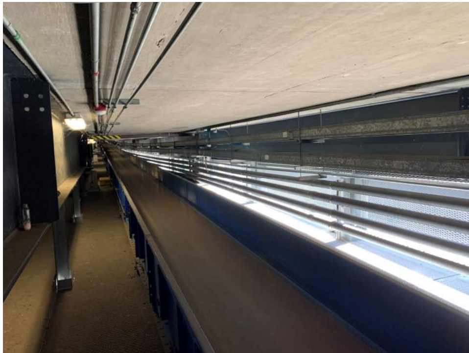
Photo 8 – Overview of Airside E Guideway baggage area below walkway.
