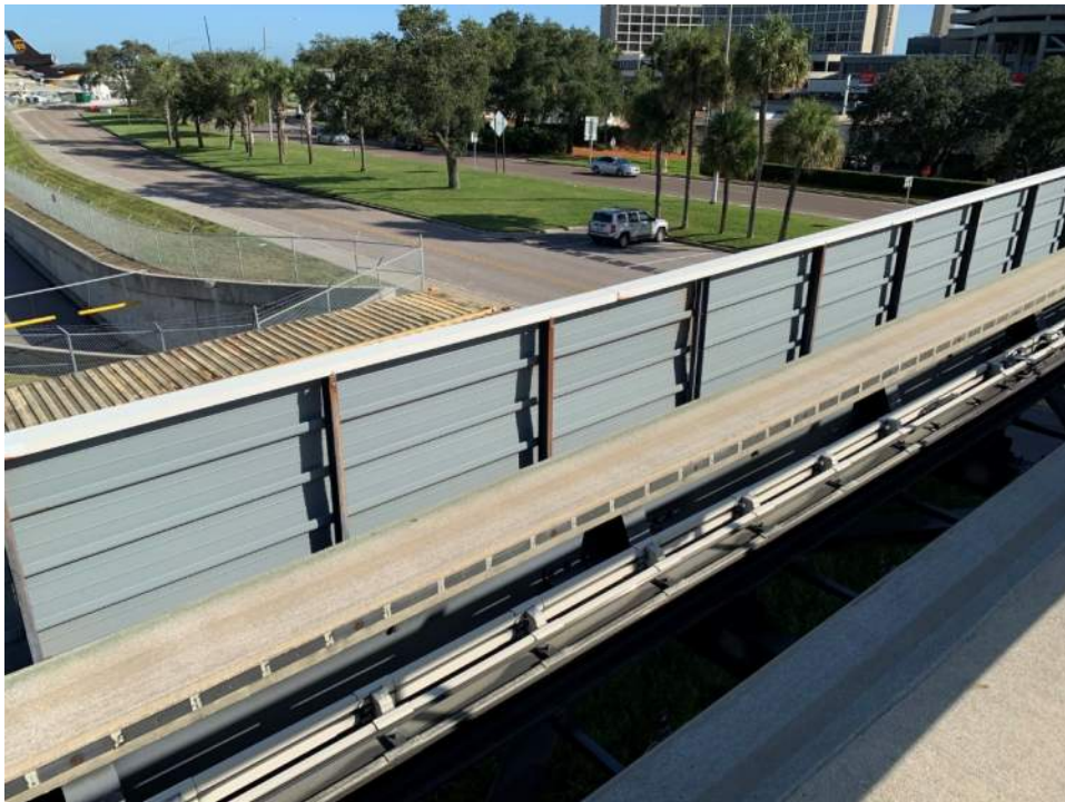
Photo 6 – Overview of Airside E Guideway running surface.
