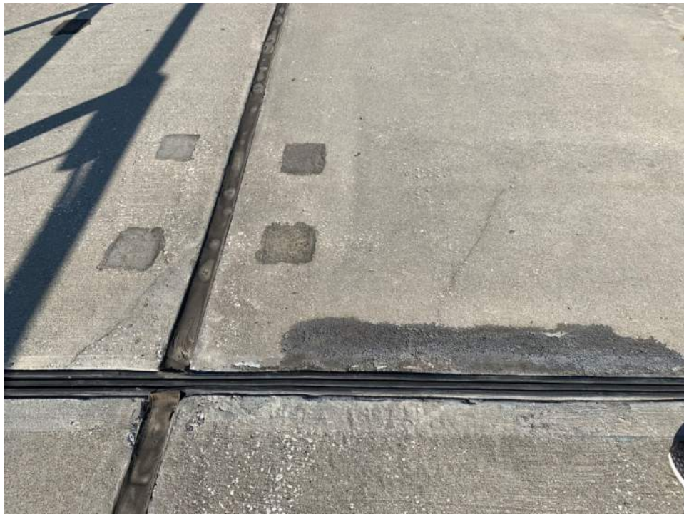
Photo 4 – Typical Airside A-Sort Guideway expansion joint detail.
