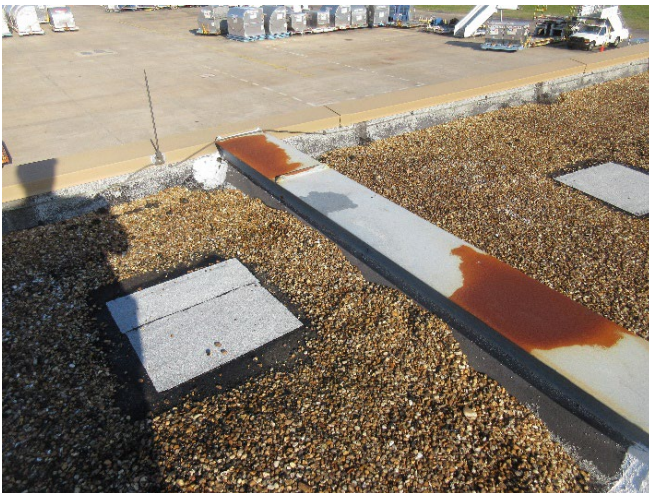
Photo 7 – Typical expansion joint.
