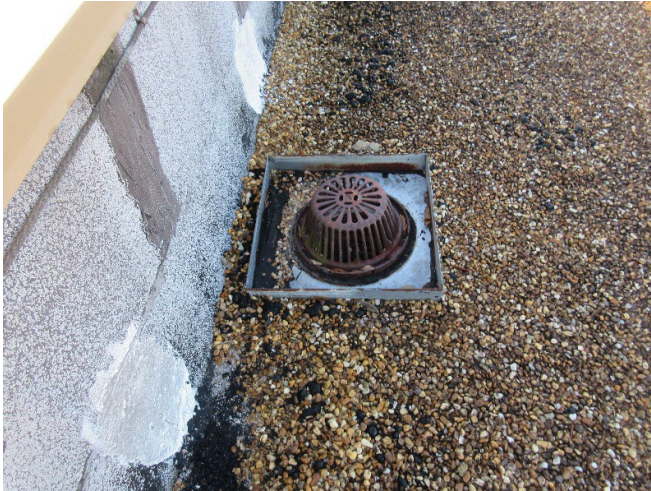
Photo 9 – Typical overflow drain.
