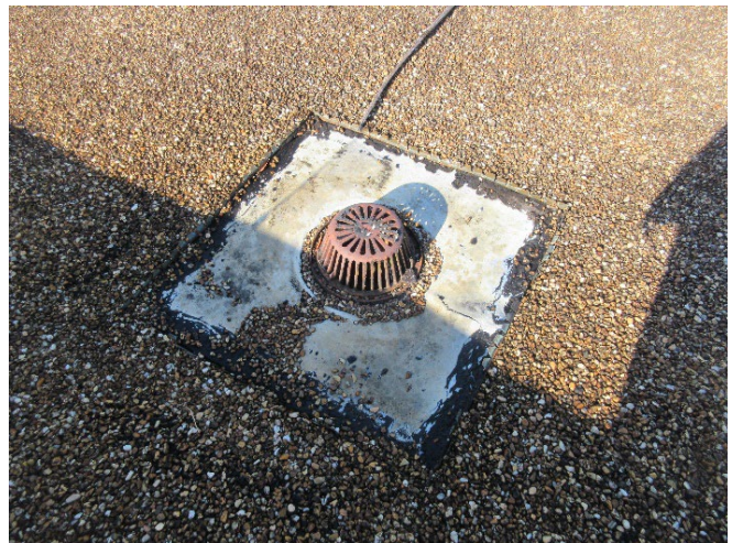
Photo 8 – Typical roof drain.
