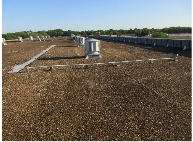
Photo 2 – Typical roof configuration.
